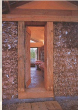
Timber frame w Recycled fibre infill
