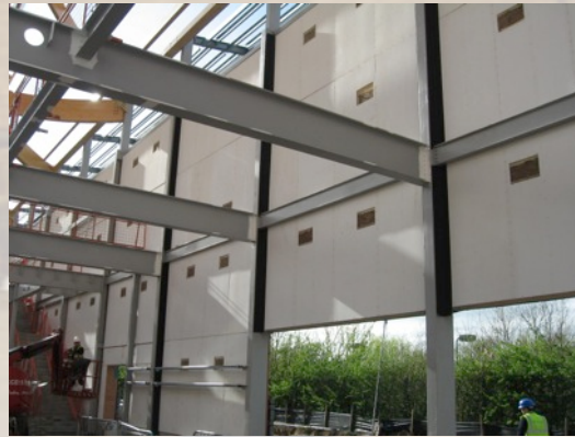
M & S panel installation
