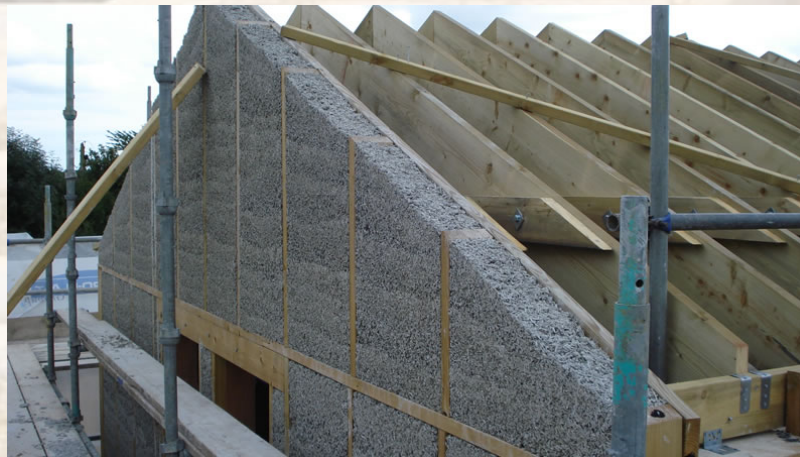
Hempcrete block winery, France
