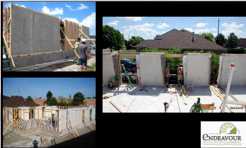
Endeavor centre prefab strawbale by Naturebuilt, Ontario
