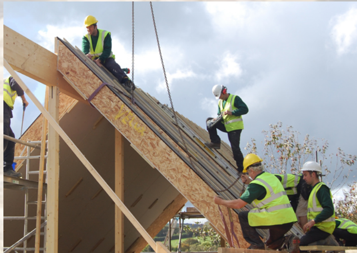
Site construction of school by Ecofab
