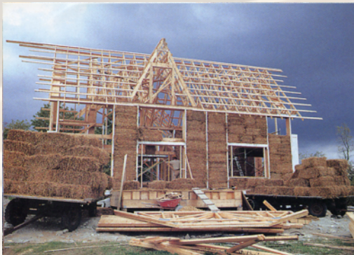
Timber frame w Strawbale infill
