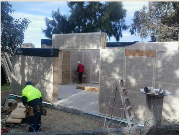
Sit-ups prefab strawbale construction by Huff & Puff, Australia
