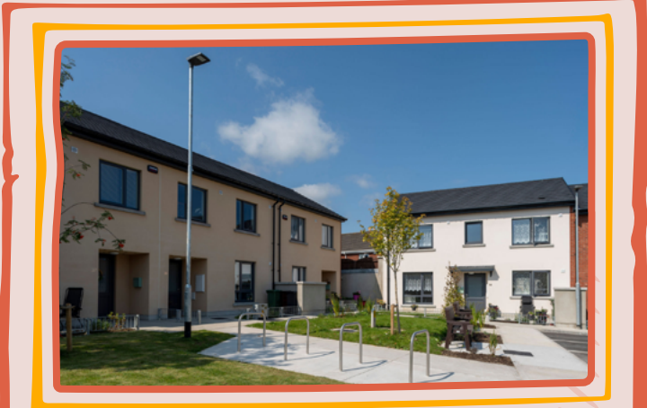
Kilbride Court (Bray) - 40 units - Wicklow City Council This the first multi-units development to reach gold standard
