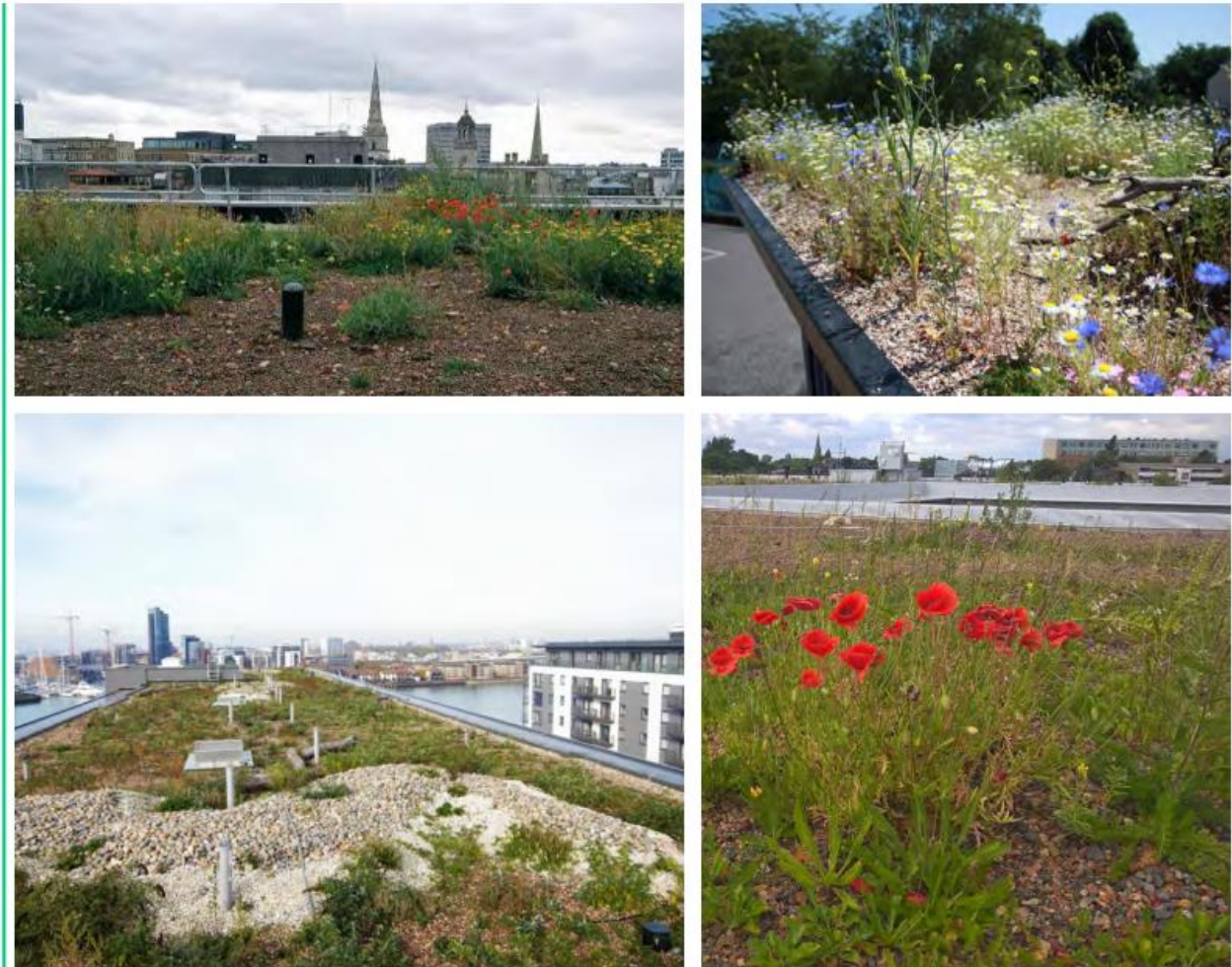
Figure 11 Example substrate types and planting variation on biodiverse living roofs
