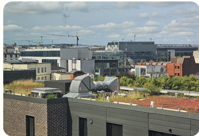
Figure 2-6: Existing Space in the 1 WML Roof Picture taken by Neil Menzies, 2024
