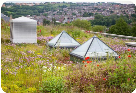
Figure 2-2: Example of semi-intensive green roof Source: Universal Floral (2025)
