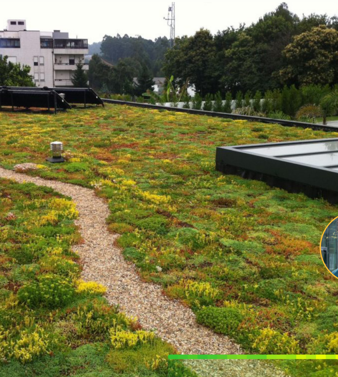
Figure 2-1: Example of semi-intensive green roof, Portugal Source: European Federation, Green Roofs & Walls (2025)
