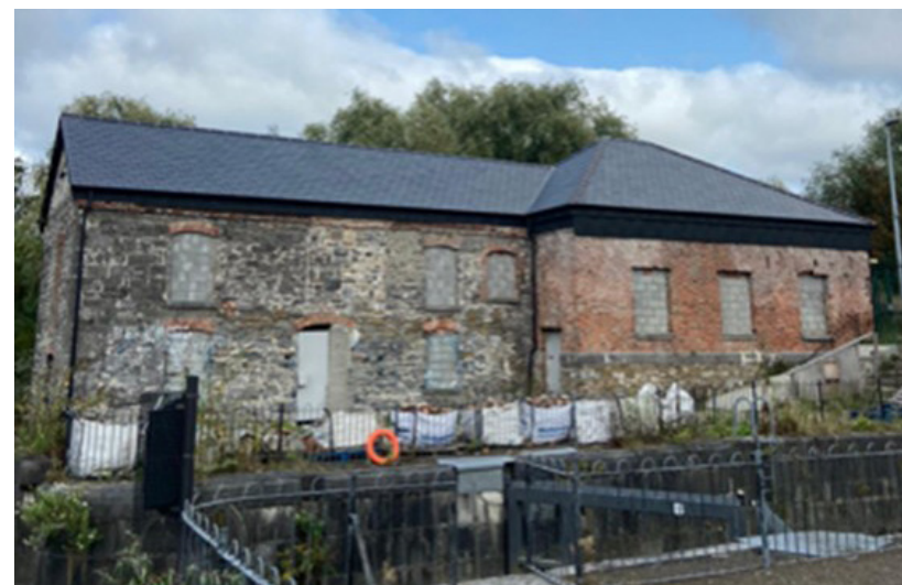
Canal Harbour Building (2,000 bricks from Opera project utilised for repairs)
