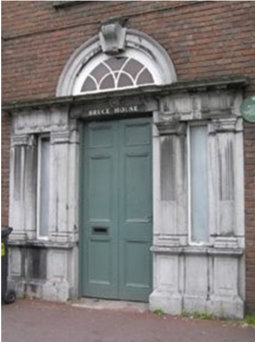
Limestone door recovered for reuse
