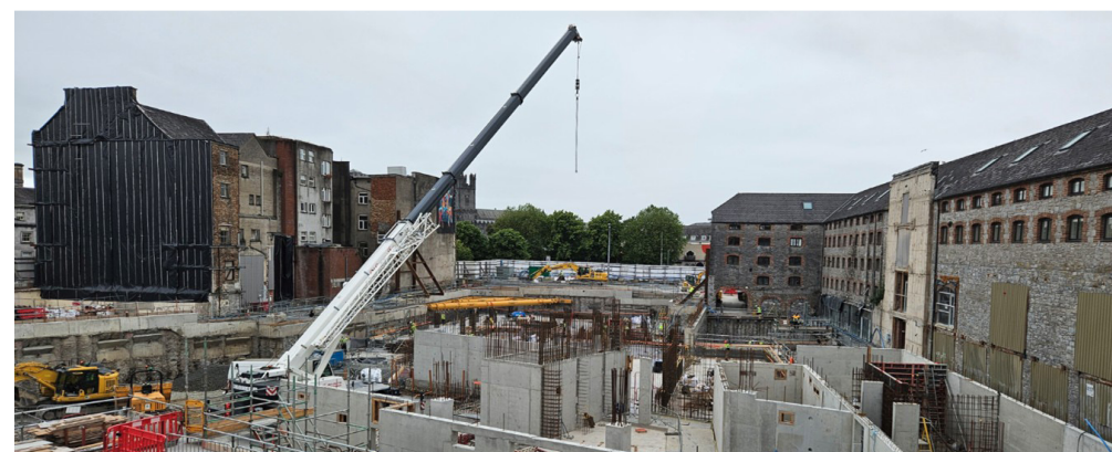
One Opera Square (under construction)
