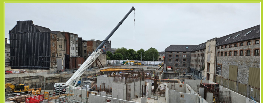
One Opera Square (under construction)
